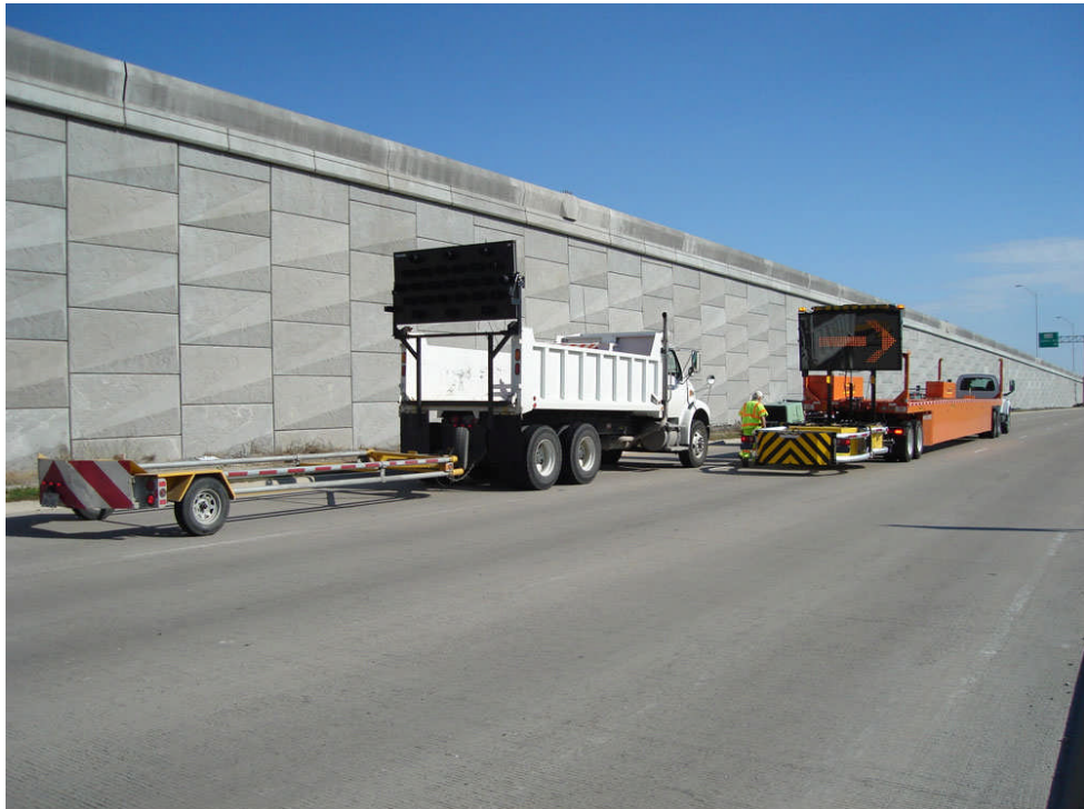
Double lane closure with additional TMA blocking entry to left lane
