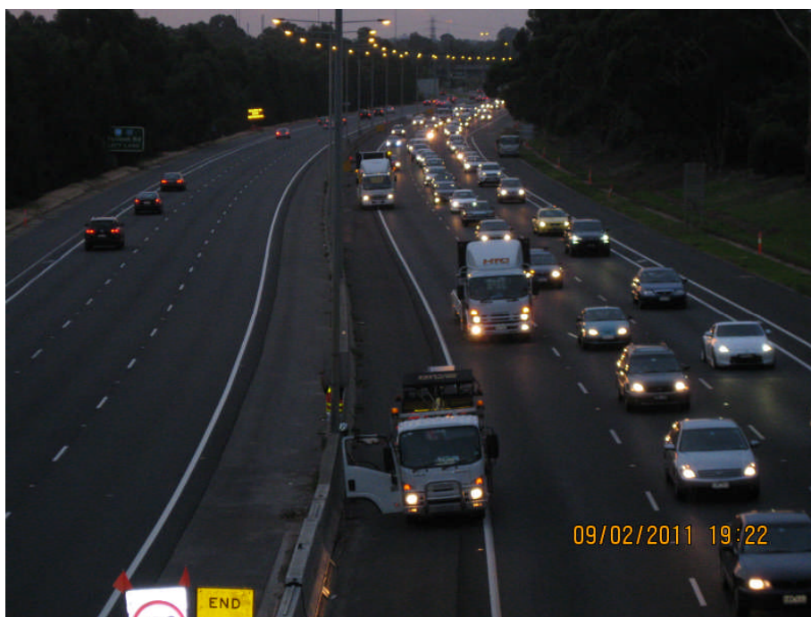
View from traffic management vehicle end of works
