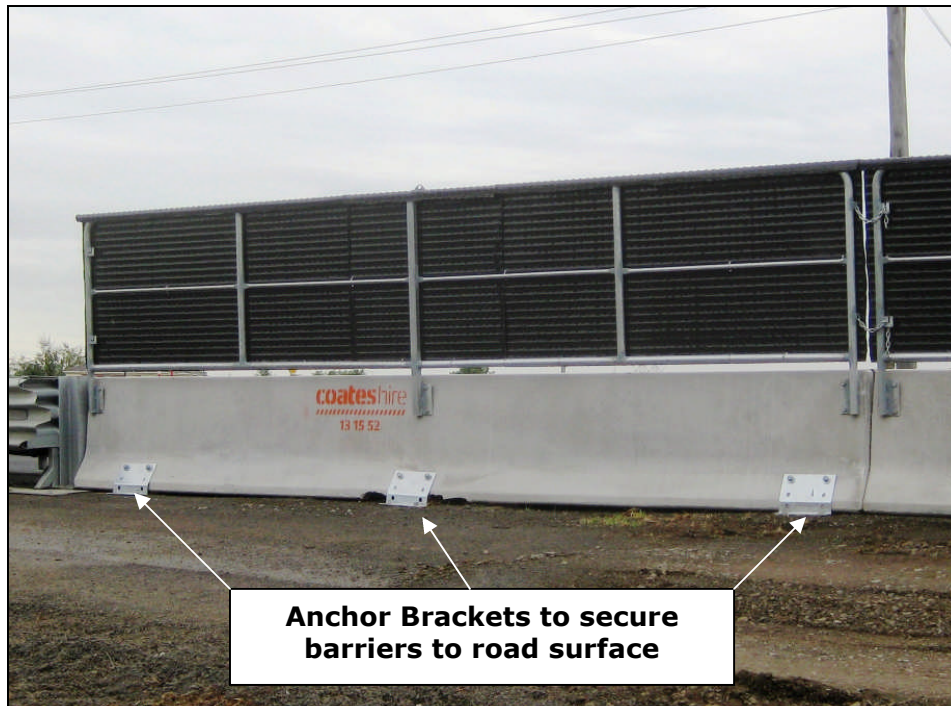
A Quadguard CZ installation showing the required anchoring brackets for the first concrete barrier unit
