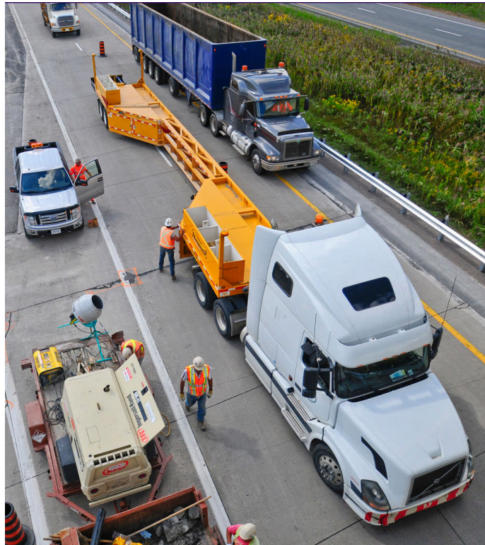
Emergency lane and lane closure
