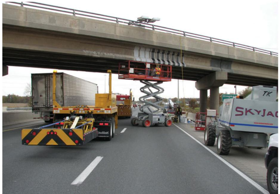
**Mobile Barriers 1:** The MBT-1 mobile barrier with scissor lift being used near London in Ontario, Canada
